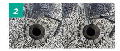
3. PLACE THE DRAIN COVER BACK ON TOP OF THE DRAIN AND TIGHTEN THE NUTS, SECURING THE DRAIN TO THE ROOF.
